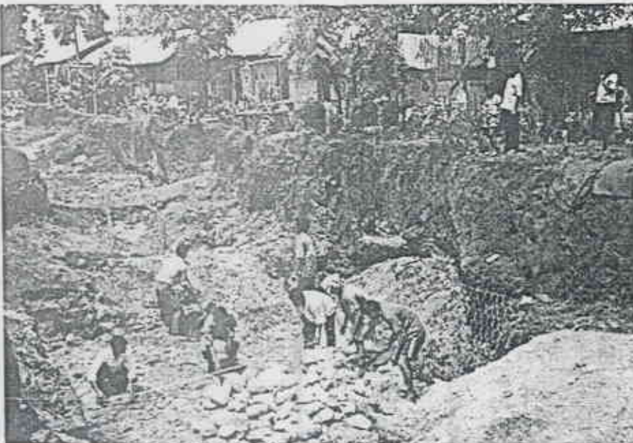
c. GULLY EROSION CONTROL AT BHUTANESE REFUGEE CAMP
