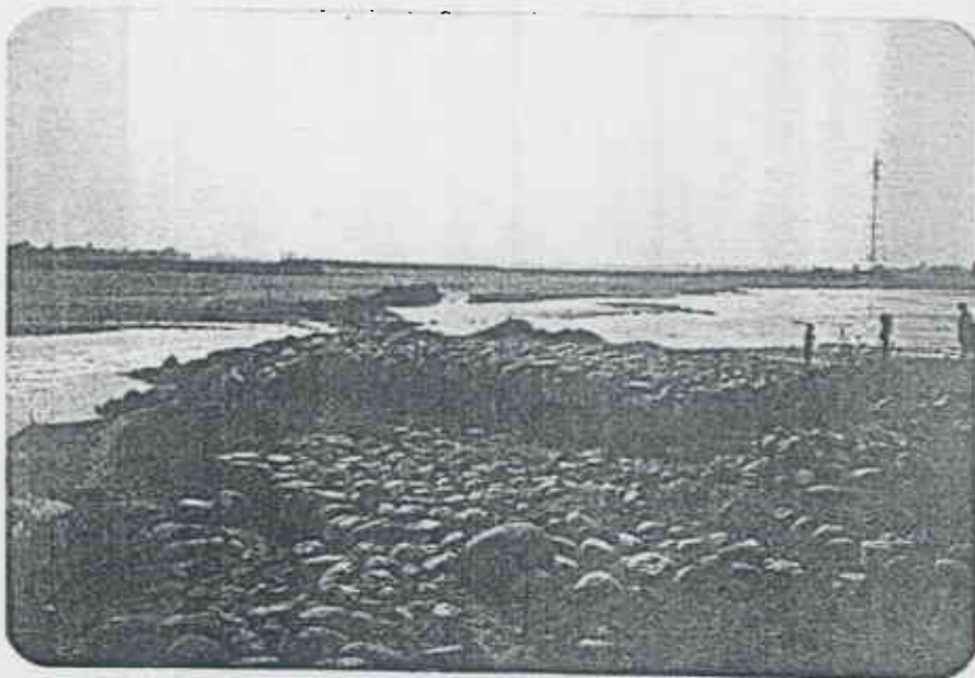
b. RIVER BANK PROTECTION AT REFUGEE AFFECTED AREA
