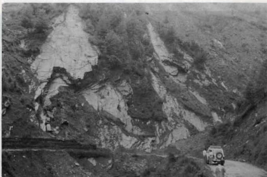
Plate 21: The plane rockslide on the Tistung Formation, near Kulgaun, Km 64, on the Tribhuvan Highway. View towards the south-west
