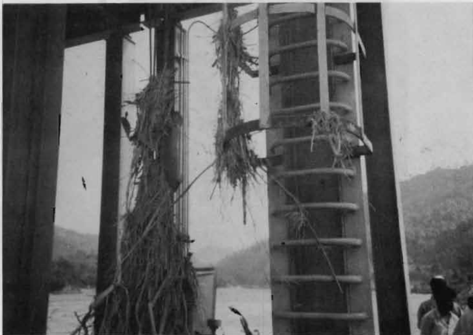
Debris entangled above the gates
