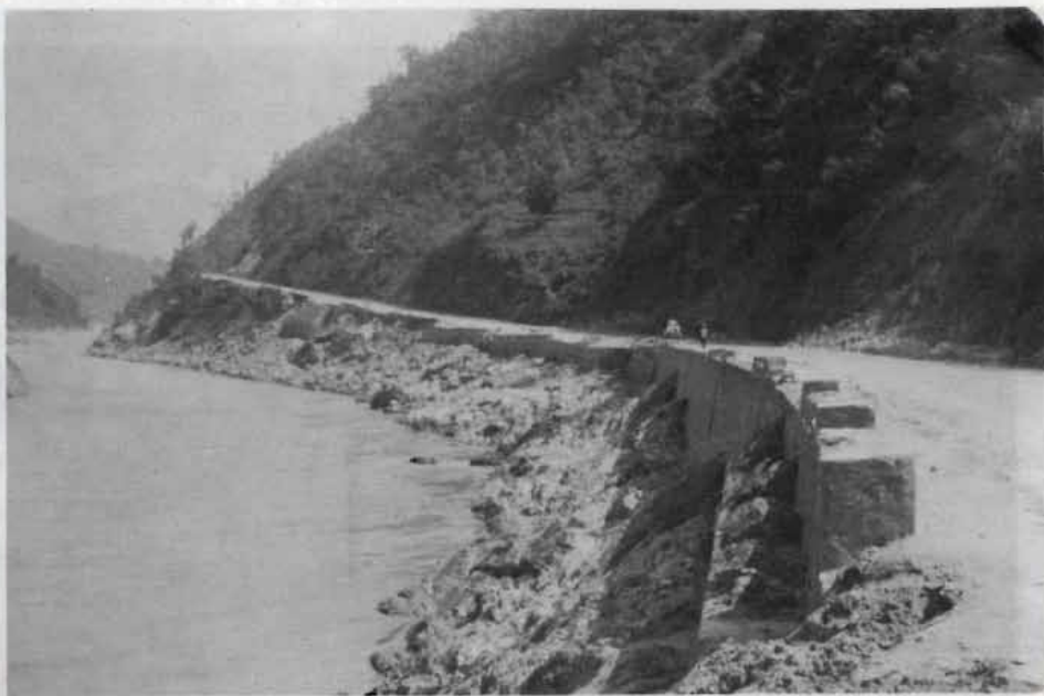
Plate 31: The Prithvi Highway to the east of Jogimara. Notice the thick silt and sand deposits on the road and washed out retaining walls. View towards the south-east
