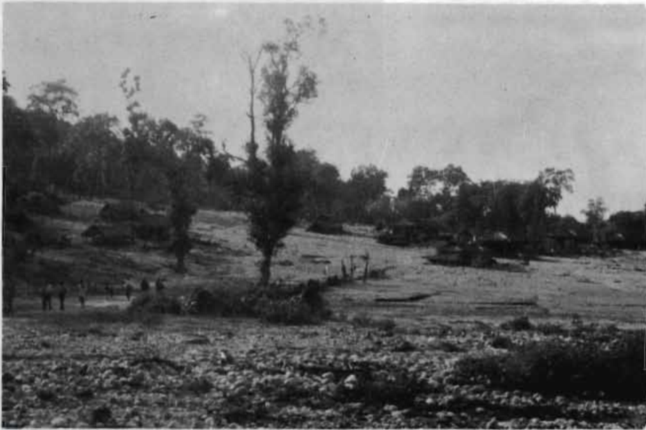
Plate 51: Sheet flooding and debris flow in the southern part of Karaonje. Notice that the damaged village is in the middle of the fan. View towards the north
