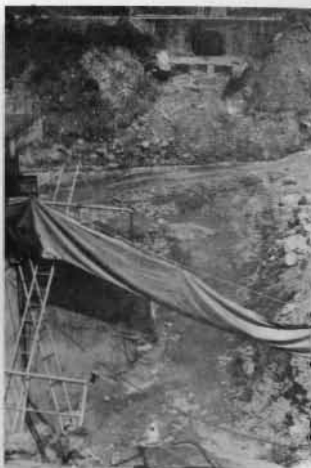
Plate 62: The outlet portal of the Kulekhari I tailrace tunnel damaged by the debris flow from the Mandu Khola. Notice also the damaged intake canal of Kulekhari II. View towards the north
