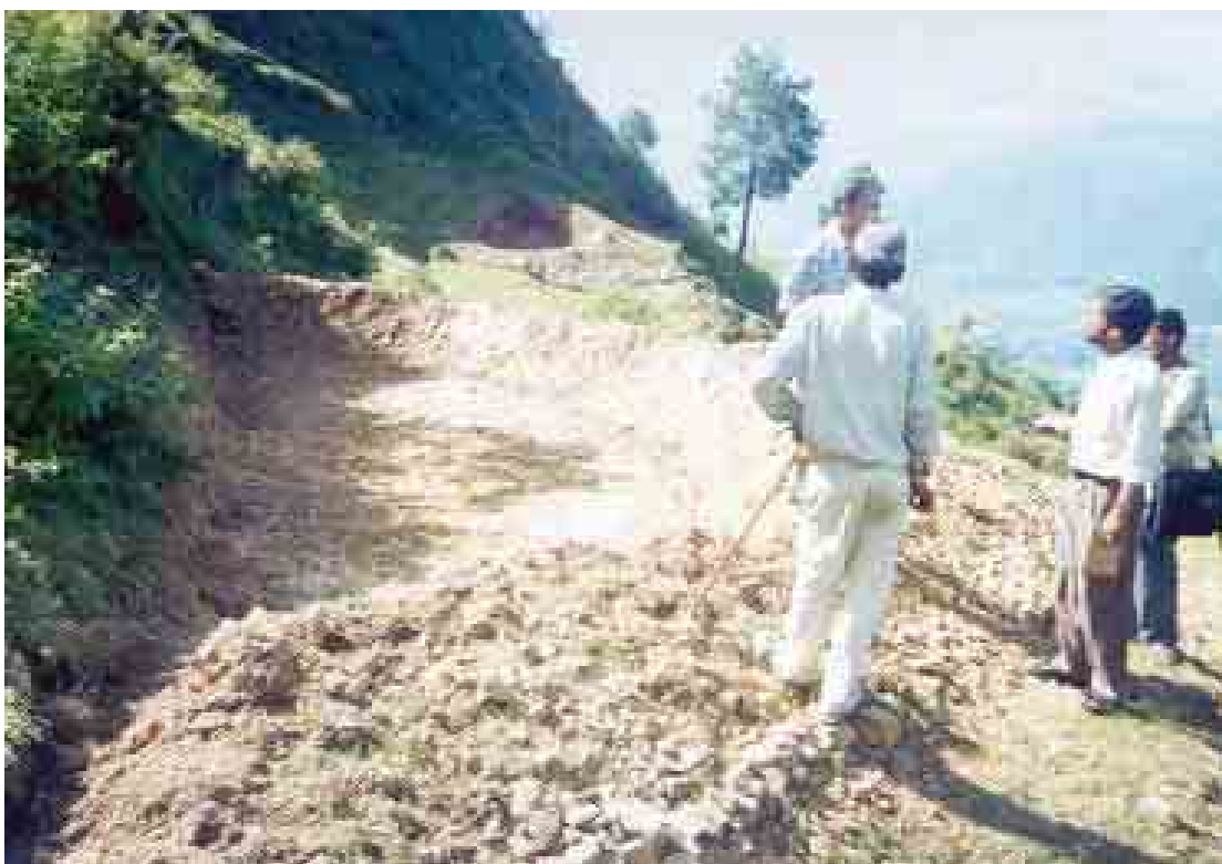
Figure 4.9: A micro-reservoir for recharging the traditional spring in Bajeena, Uttarakhand
