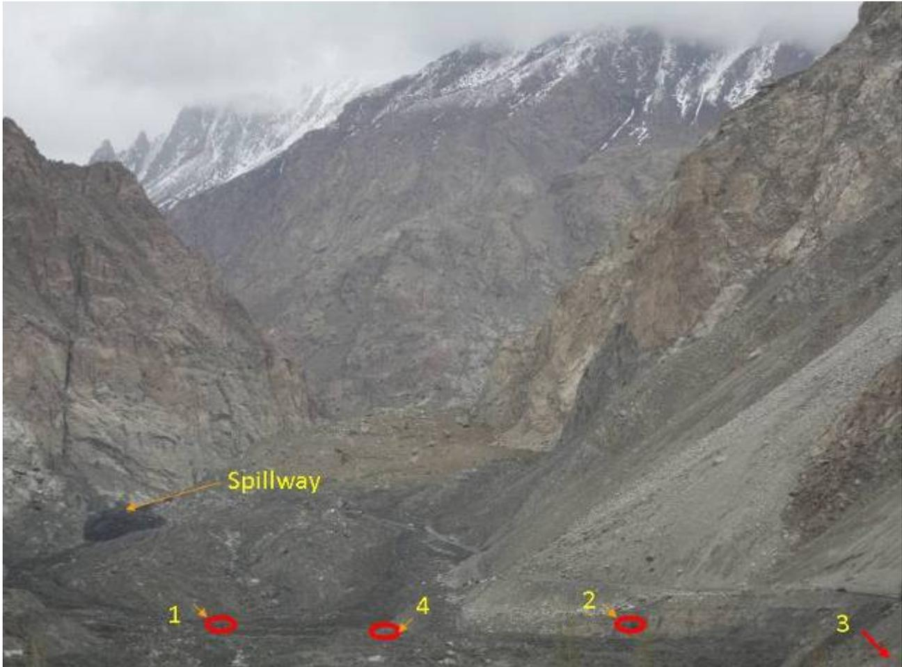
**Figure 11: Seepage points at the toe of the dam (web source).**
