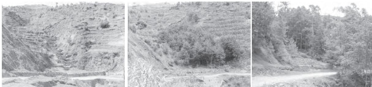
Photo 5, 6 and 7 : Treated landslide in Kunchhal, Bajrabarahi-3, Makawanpur in 1989, 1995 and 2008
