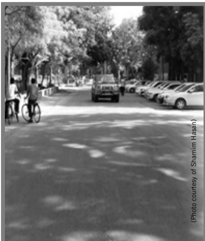
Strip of waste plastic mixed bitumen road at BUET, Dhaka
