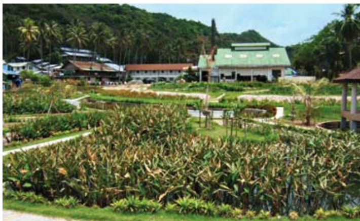
Constructed wetlands on Phi Phi Island, Thailand, which are used for treating wastewater from hotels and restaurants. (Photo: A. Morel)
