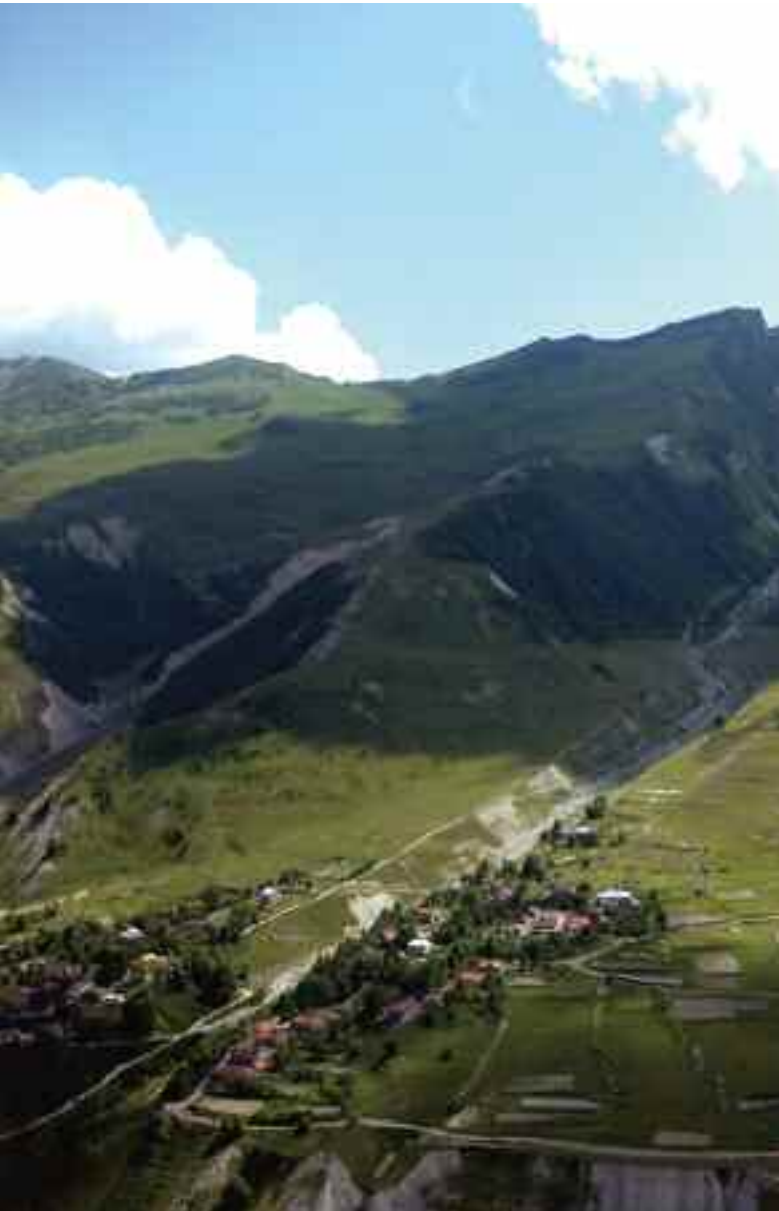
Figure 1: Erosion and settlement. Photo: Maia Akhalkatsi.
