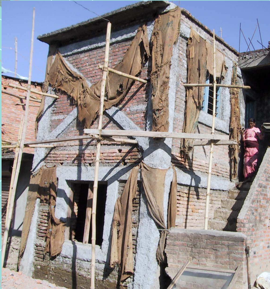
Bracing to increase lateral strength of wall
