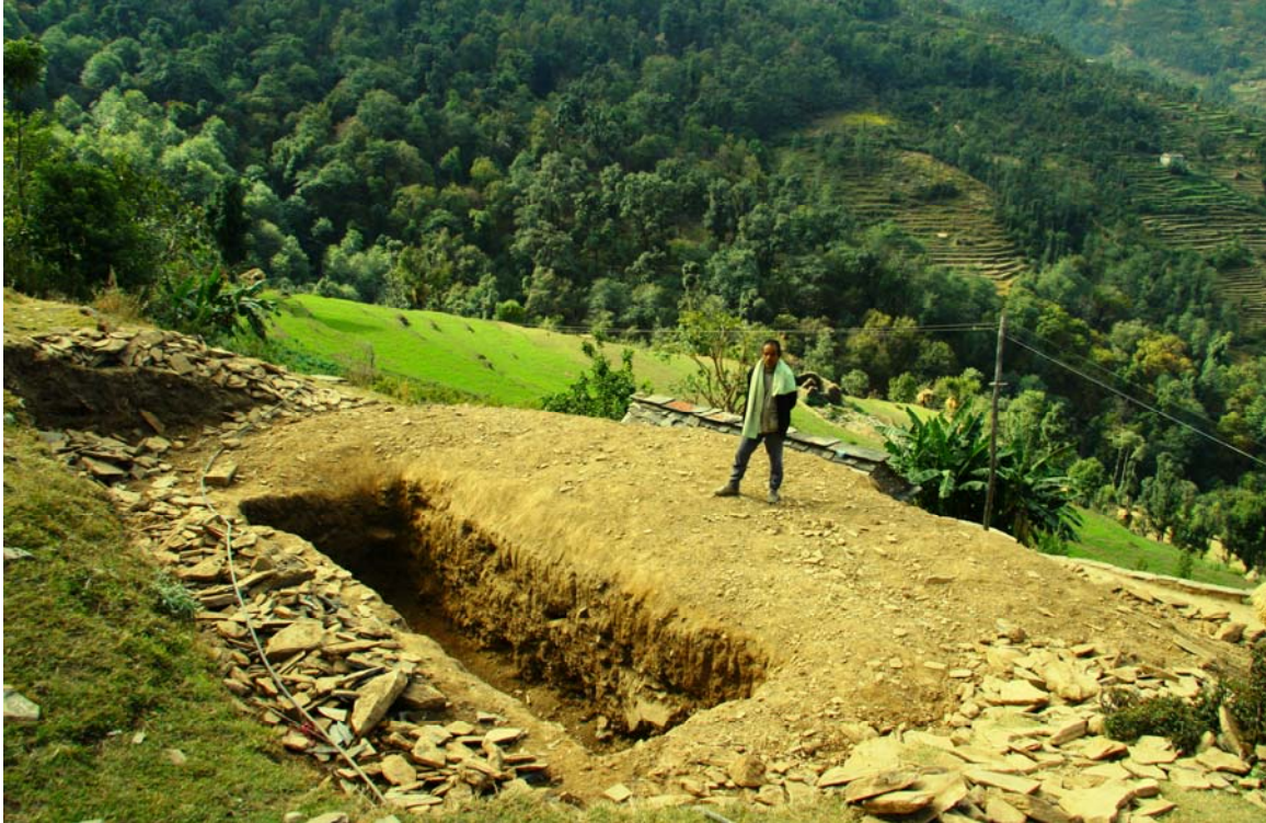
Photo 3: Rain water harvesting system being initiated by SABAL Project in Accham. Rain-water harvesting systems like these are very cost effective to build yet has little capacity and cannot provide adequate irrigation facilities to a large number of households. Typically, a system like this is only adequate to provide irrigation facilities to 7-8 households for a small plot of land.
