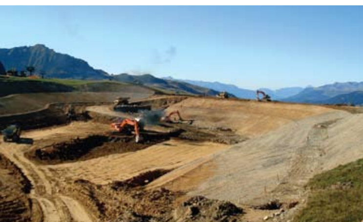
Preparatory works for the construction of an artificial reservoir (125,000 m 3 ) at Ariondaz (2,500 m) to store water for artificial snow making for the ski lifts of Courchevel, French Alps. Photo: Benjamin Damelet
