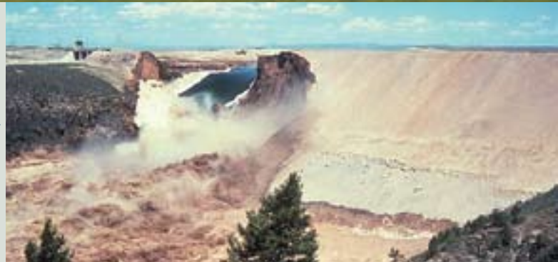
The collapse of the Teton Dam on June 5, 1976 released nearly 300,000 acre feet of water, killed eleven people and caused nearly a billion dollars in damages to the farmland and towns downstream.
