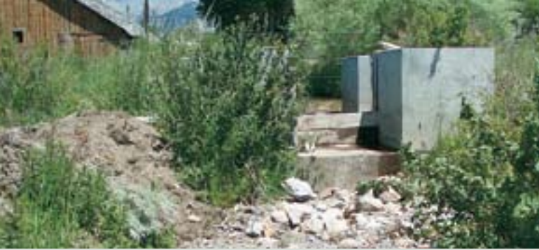
Left: Badger Creek diversion structure removed all flow from the lower stream reaches during the summer, effectively dewatering the natural channel and cutting off access to spawning and rearing areas for fluvial fish.
