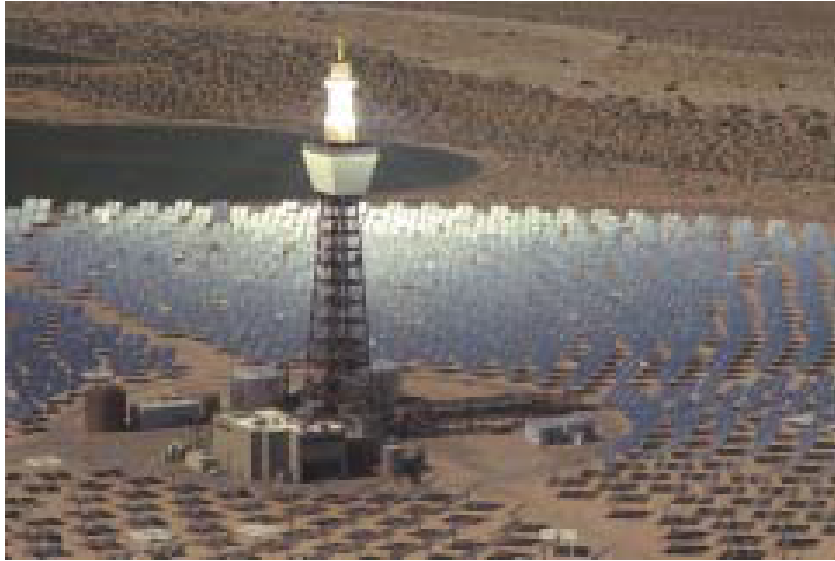
Figure 3.2: A picture of Solar Two, the prototype power tower. Some 1,926 heliostat mirrors are used to produce 10 million watts of electricity. Source: Sandia Laboratories.
