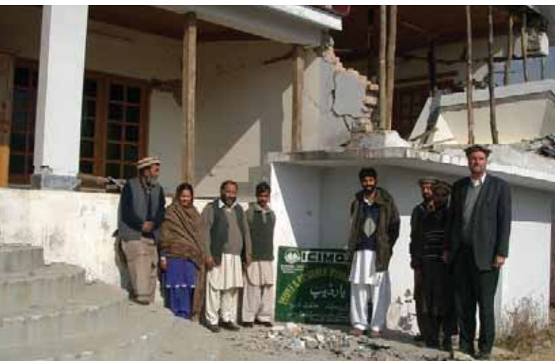
After the earthquake in October 2005, Hilkot, Pakistan. Photo: ICIMOD
