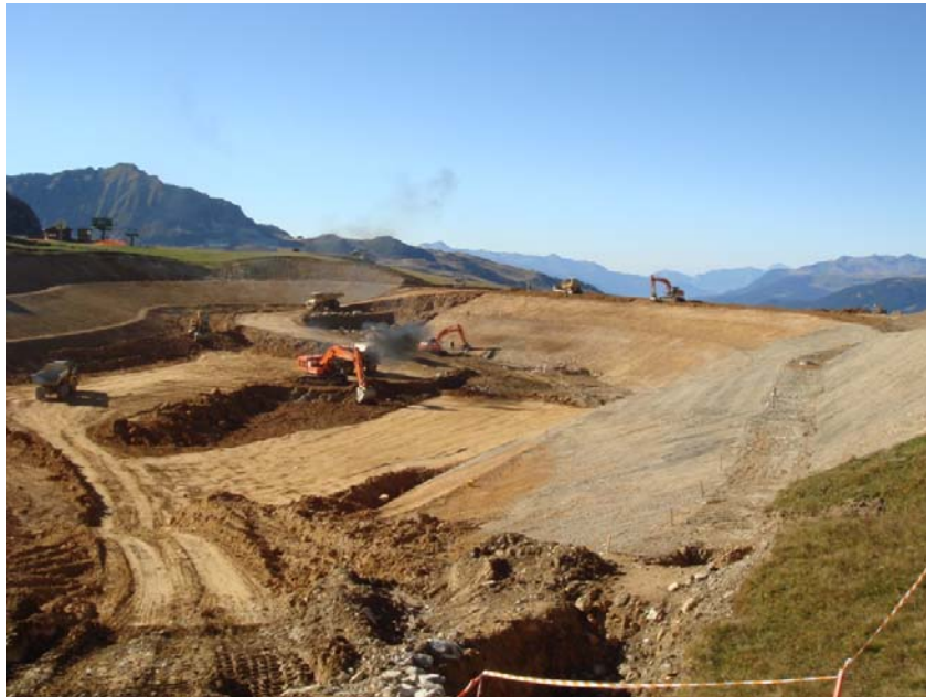
Preparatory works for the construction of an artificial reservoir (125 000 m 3 ) at Ariondaz (2500 m) to store water for artificial snow making for the ski lifts of Courchevel, French Alps. (Bejamin Damelet 2007)
