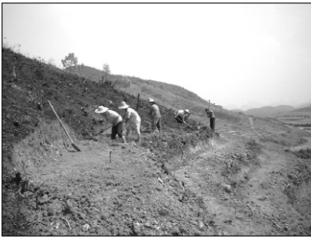
Figure 9.6 Villagers terracing the land to establish an orchard Photo: Yuan Juanwen.
