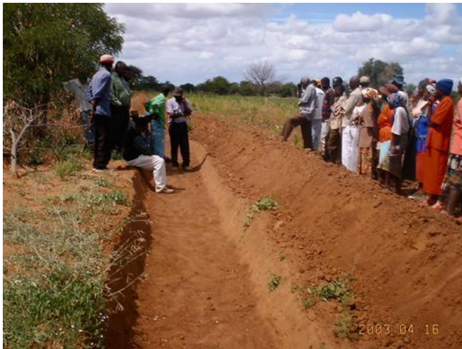
Figure 2: Complete dead level contour ready to harvest water Credit: Practical Action
