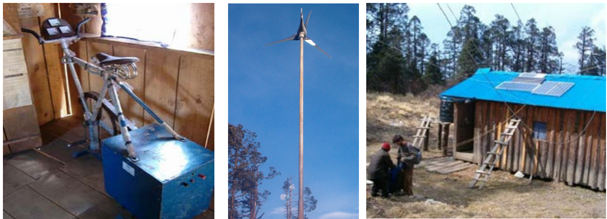
Power Generation Equipment (from left to right) a bicycle generator, wind generator, and roof-mounted solar panels
