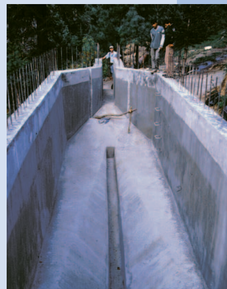
FIGURE 3 Desilting tank in Kothi. The tank ( 34 \times 2.5 \times 1.5 m), made of reinforced concrete, desilts water on its way to two 100-kW turbines. (Photo by author)
